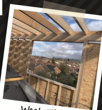
Week Three New dormer going up
