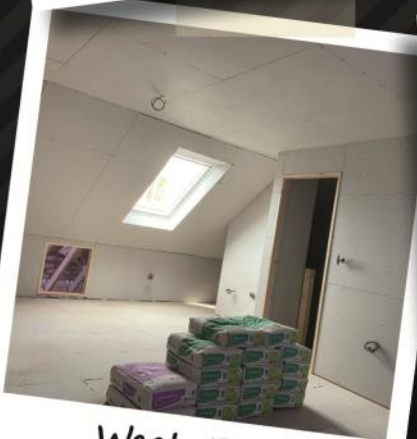
Week Five Internals being finished
